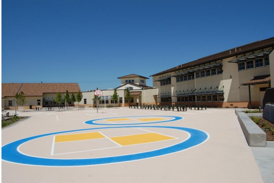
Figure 6. Reflective coating at Martin Luther King, Jr. Elementary School
